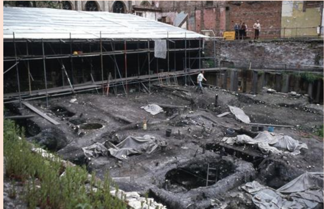
Photo of Coppergate excavation site
