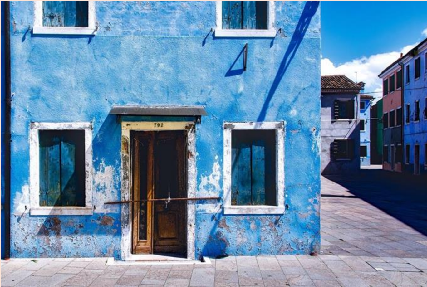
Front of a building and side street
